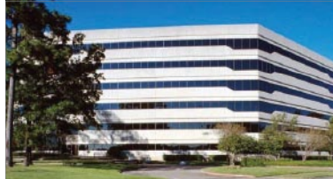
Bridgestone I* 2600 N. Loop Freeway Northwest Submarket
